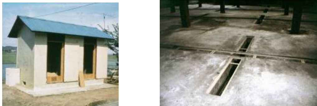
Figure 22: Korean low-temperature in-bin drying and storage system (IBDS) at farm level (left), aeration ducts in a large storage system (right)
